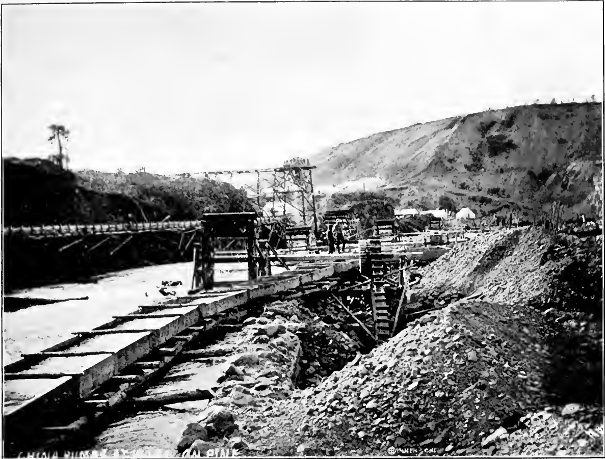
CHINESE PUMPS ON PINE CREEK—ATLIN M. D.
